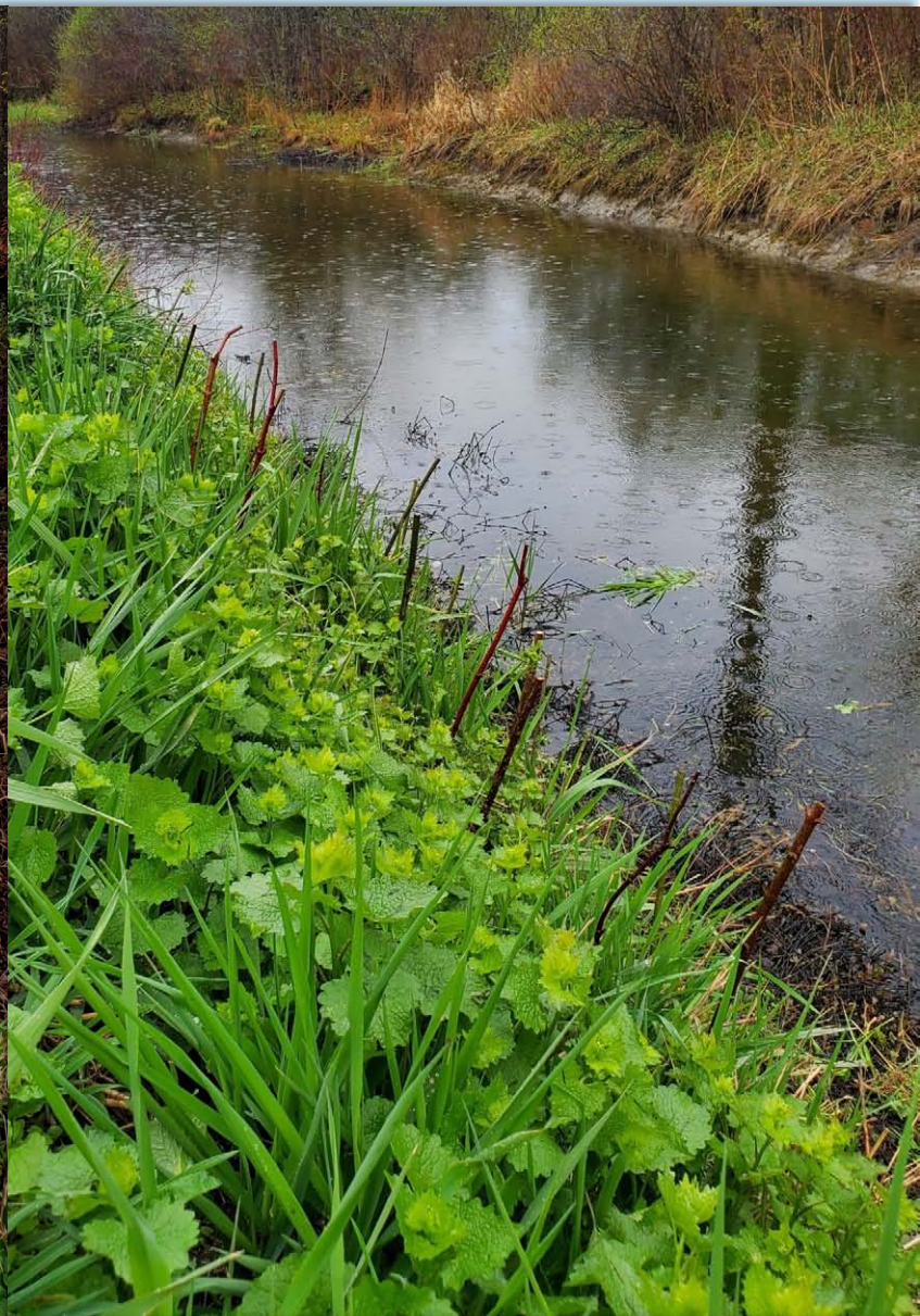
After live stake installation
